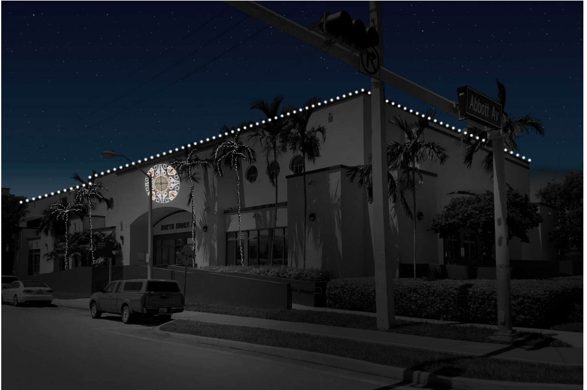
North Shore Park - Lights installed in October, Scroll installed in November Miami Beach / Florida
